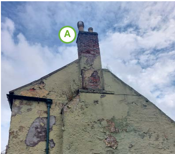
A Using raincoat repairs on a greatcoat building can lead to damp walls, as well as weathering and erosion of the core building material.
