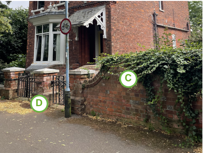
A Cast-iron railings define the front boundaries of many late 18th and 19th century housing areas. The iron industry produced a wide range of decorative cast and wrought iron railings and gates, varying in style from restrained to highly
