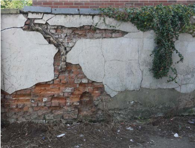
A Using raincoat repairs on a greatcoat building can lead to damp walls, as well as weathering and erosion of the core building material.
